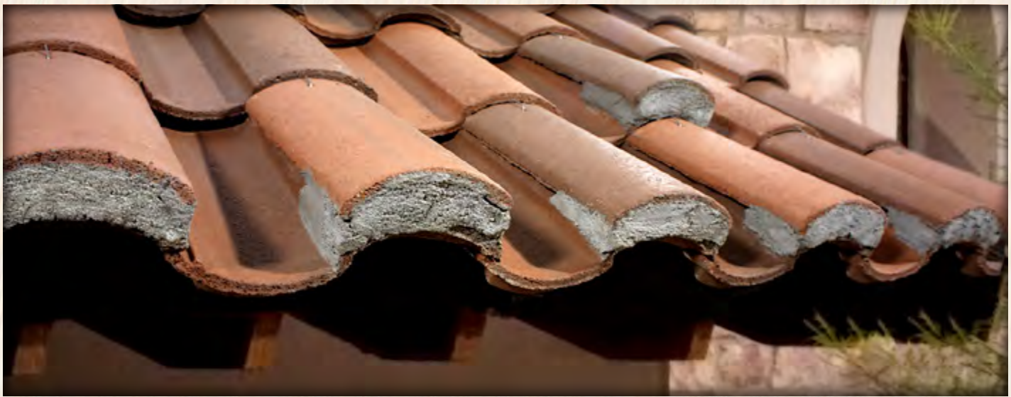
Close-Up of Boosted Eave
